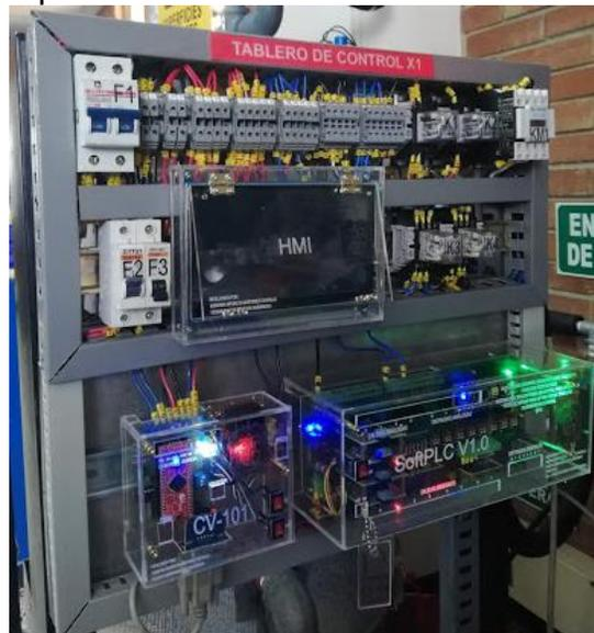
Fig 87. Tablero de control X1 Final. [Autor]
